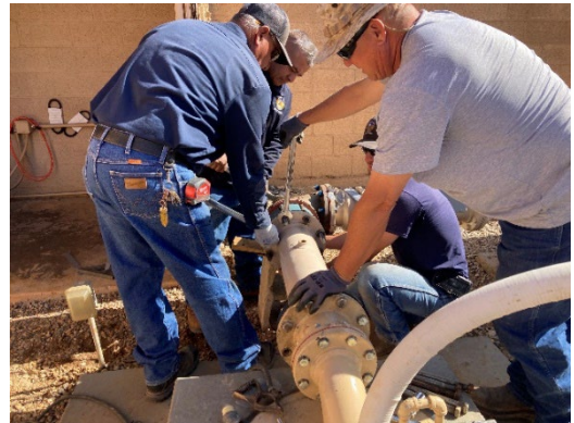
Staff replacing horizontal booster pump (left). Staff installing well discharge pipe (right).
