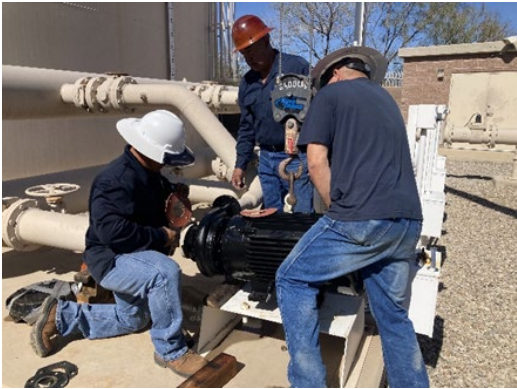
Staff replacing horizontal booster pump (left). Staff installing well discharge pipe (right).
