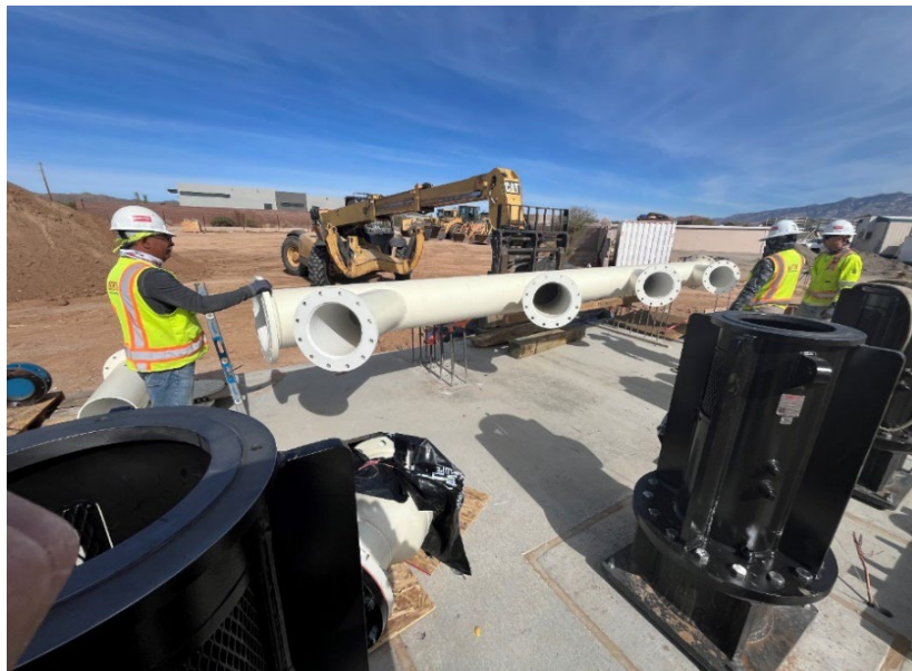
The image above shows the contractor staff fitting the discharge piping for one of the booster stations.
