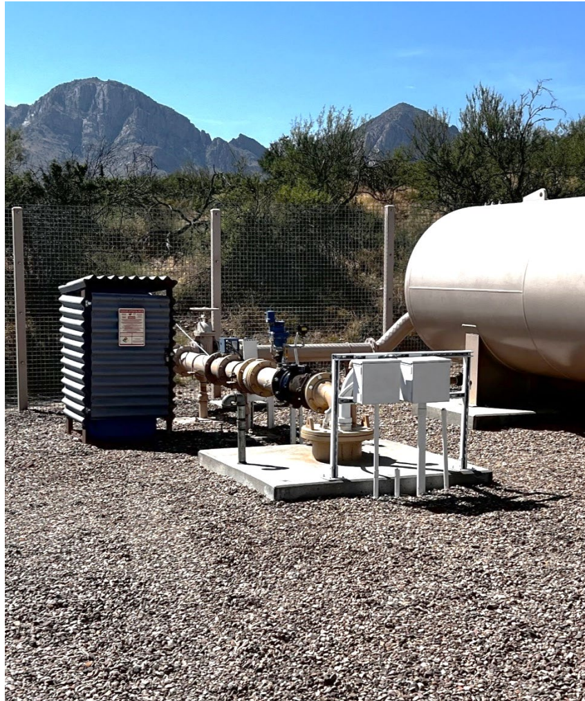
The photo above shows the completed rehabilitated of Well E-2. Work included well rehabilitation, new submersible pump, and discharge head
