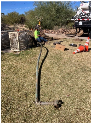
Water Distribution staff replaced a 2" copper service line at Riverfront Park (left).
