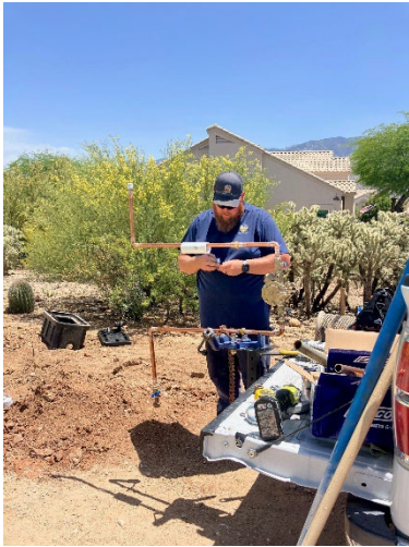
Staff repairing and testing Town of Oro Valley backflow prevention assembly. (left). Staff collecting compliance water samples (right).
