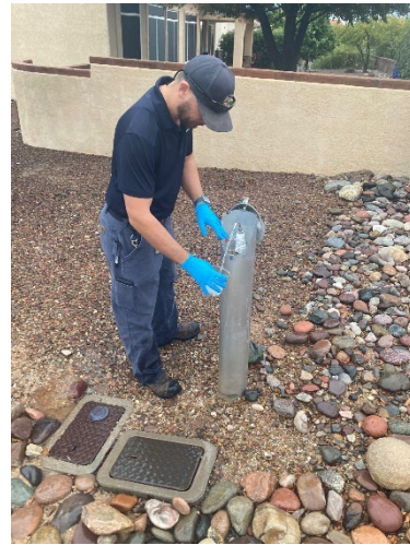
Staff repairing and testing Town of Oro Valley backflow prevention assembly. (left). Staff collecting compliance water samples (right).
