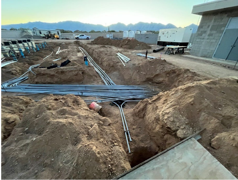
The image above shows the conduit runs from the La Canada Booster Stations to the control building.
