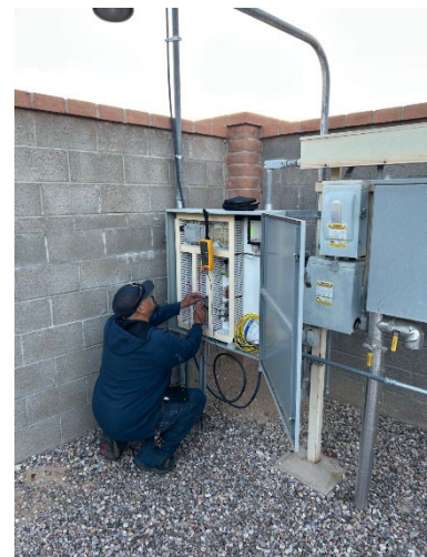
Water Control Systems staff testing PLC panel power supply(right)
